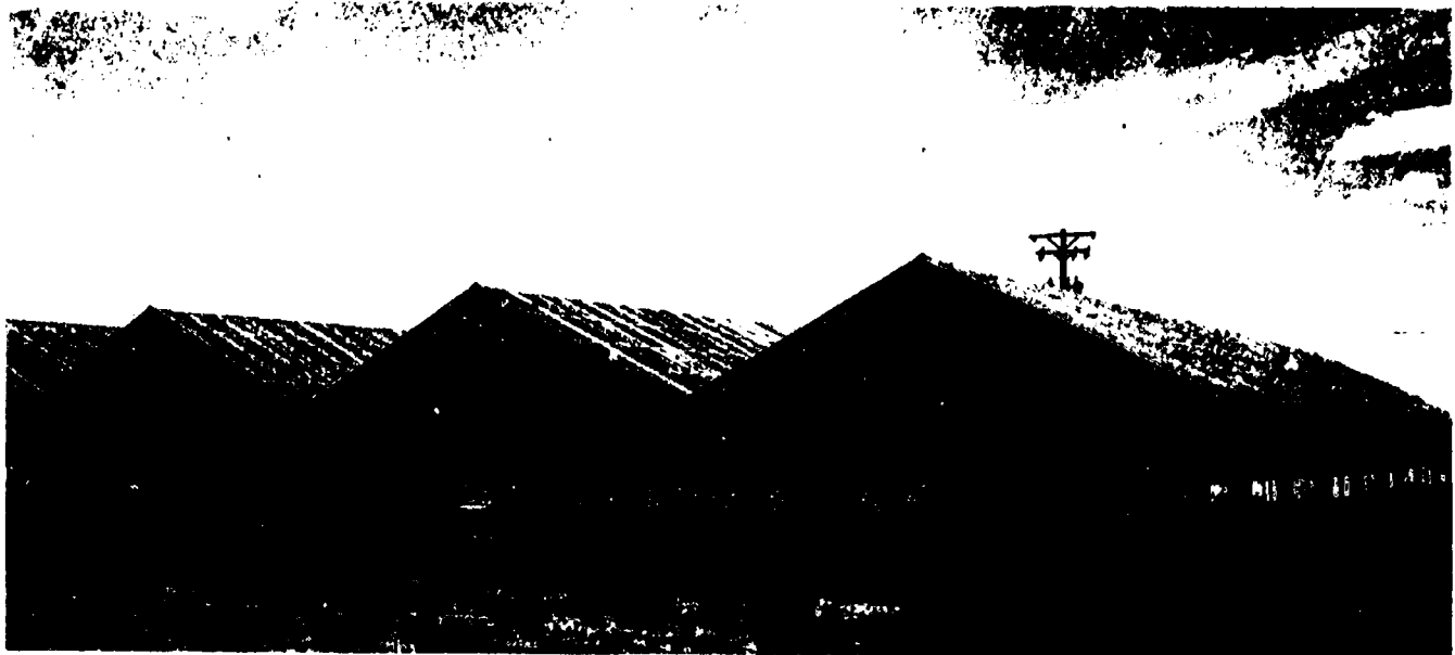
Figure 2.5 Ridge-and-furrow greenhouses, American style
