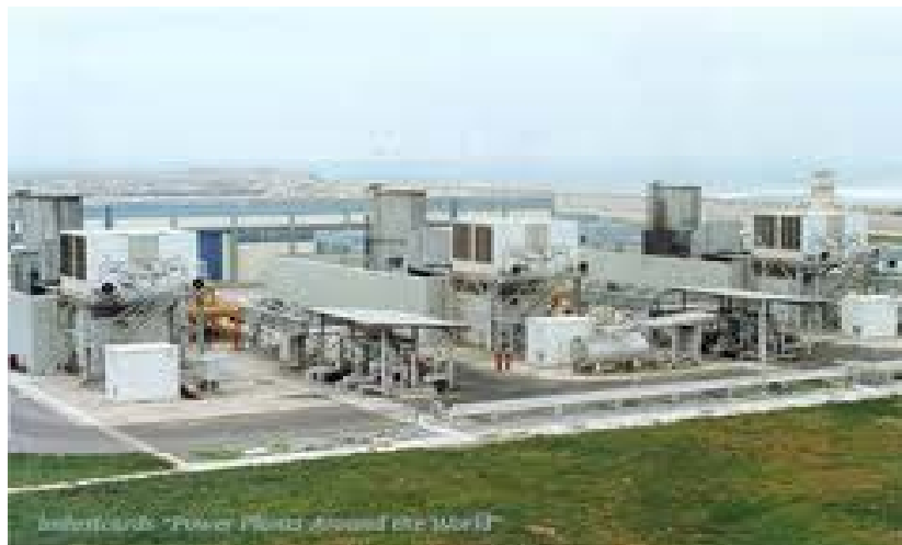
Plate 12.1. Mohammed VI Power Station in Morocco. Reproduced with permission. Image sourced from http://www.industcards.com/cc-morocco.htm
