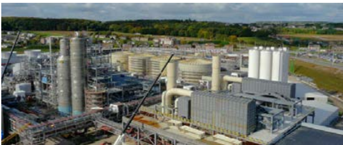
Plate 3.2. Bioethanol plant at Wanze. (Reproduced with permission of CropEnergies AG)
