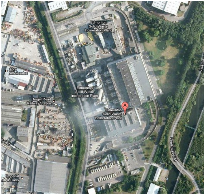
Figure 8.4 Edmonton Solid Waste Incineration Plant, London, England (Google map) (Note: type 'Incineration Plant' in Google map and it may provide some sites near where you live)
