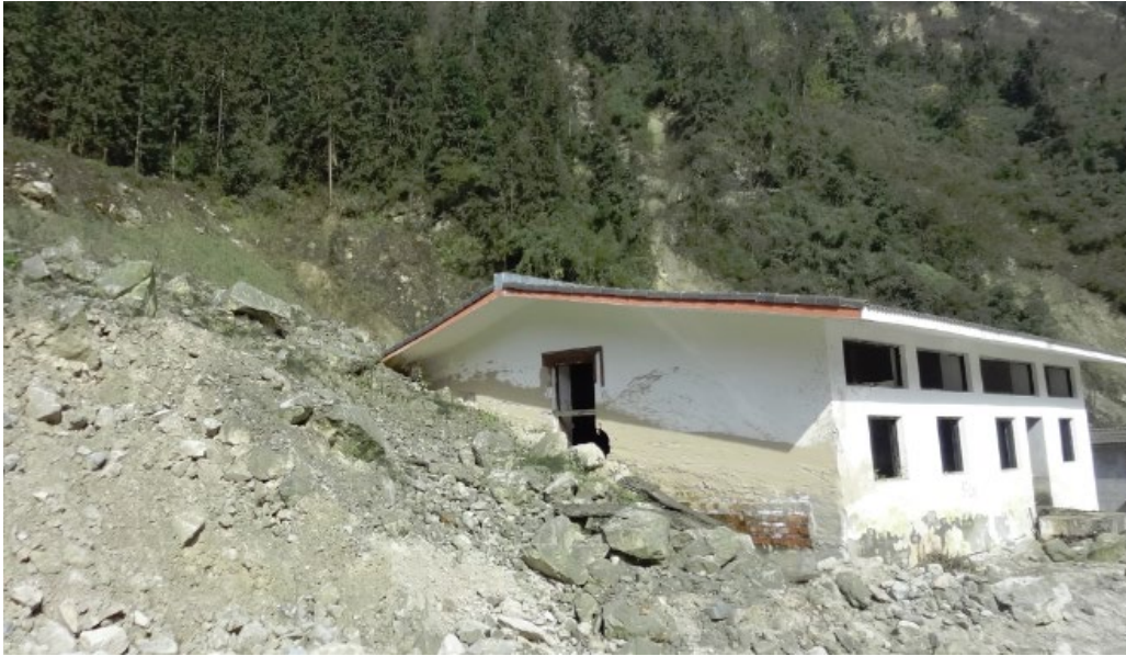
Figure 5.2 Landslide damage in Sichuan, China, 2010
