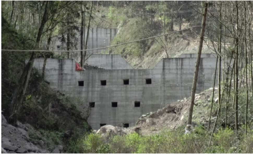
Figure 5.4 Check dam for debris flows
