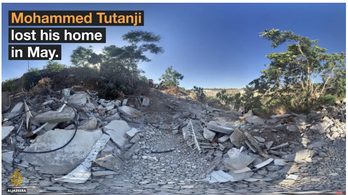
Image 2: Panoramic photograph of home demolished in May 2016.
