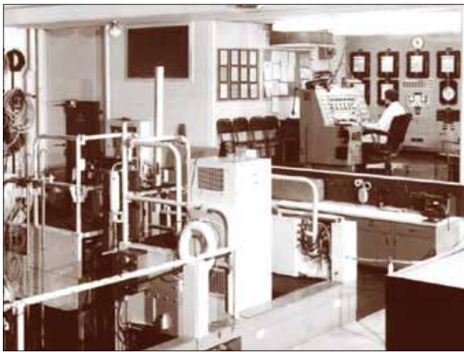
The FNR bridge and control room
