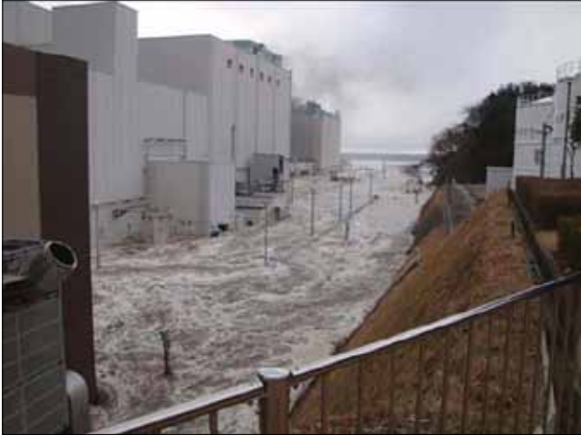
Tsunami destroys emergency cooling system
