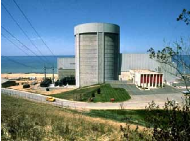
Palisades Nuclear Plant (Michigan)
